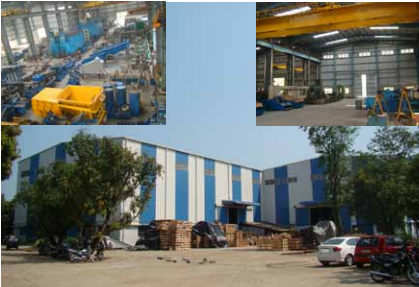
View at the inside and outside of the new Pandor factory
