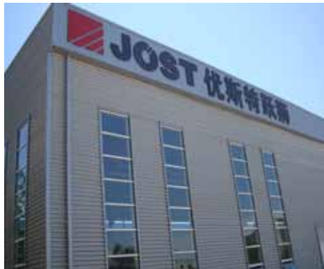
JCVT service centre north of Beijing
