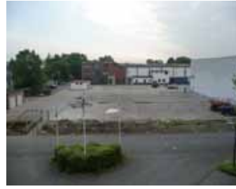
...and after demolishing of the halls.
